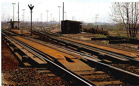
Remote controlled track retarders in the classification tracks – Mannheim switch yard
